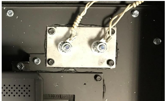
BOTH LAMP ASSEMBLIES ARE CONNECTED
