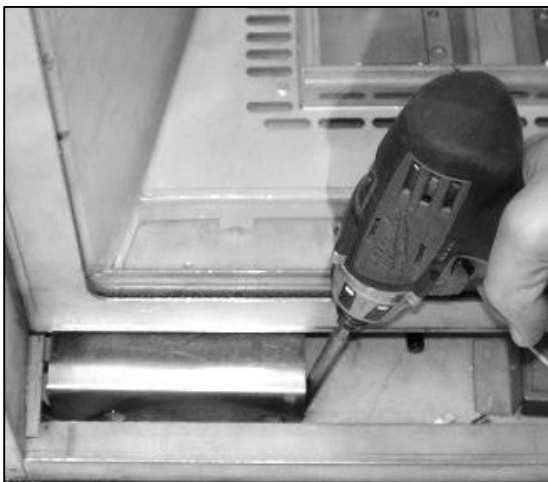
Power Vent Control Module Mounted inside fireplace.
