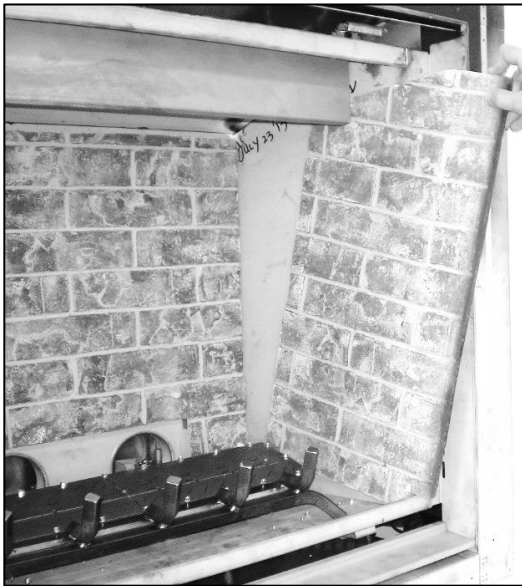
Step Three: Tilt and slide left and right Side Liners into place.
